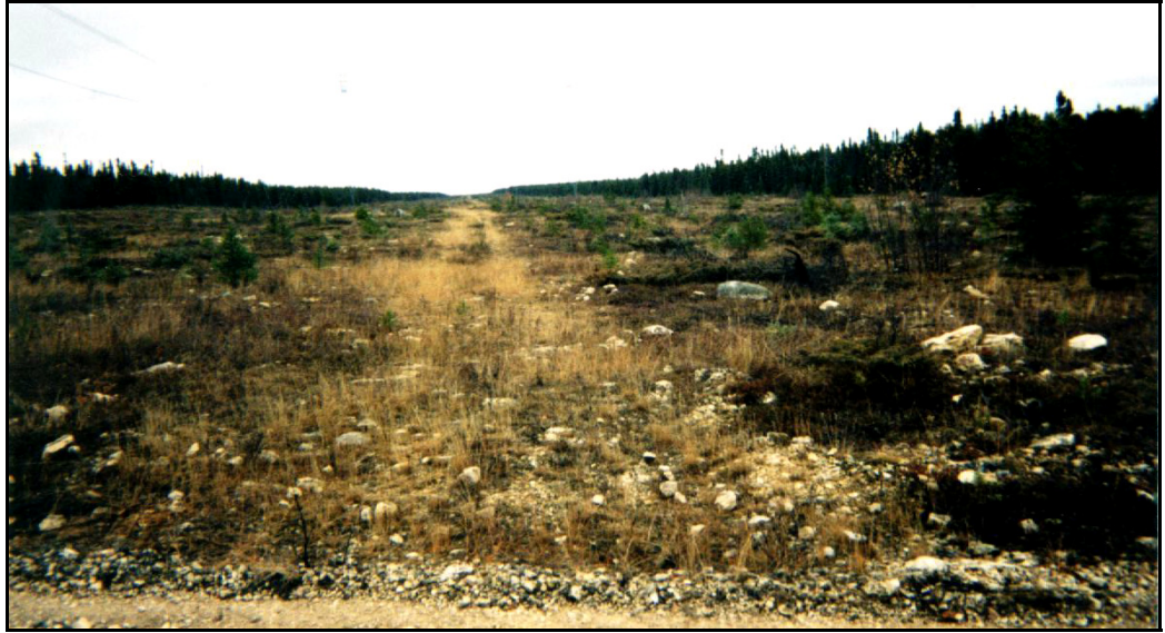
Plate 4: Example of a right-of-way for hydro-electric transmission line, showing access road.
