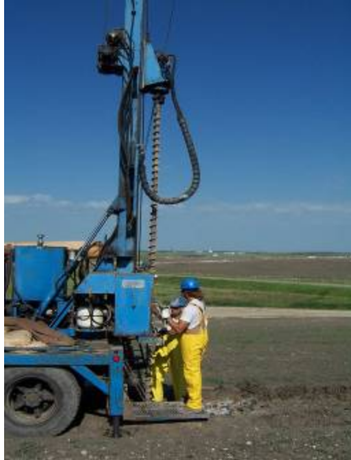
Figure 3.2 Gas monitoring probe installation on June 20 th , 2003 at Brady Road landfill
