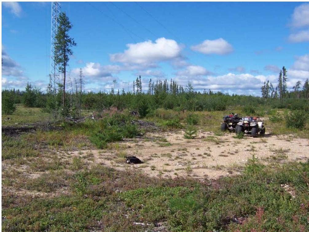
Plate 12. Hydro transmission line traversing the study area
