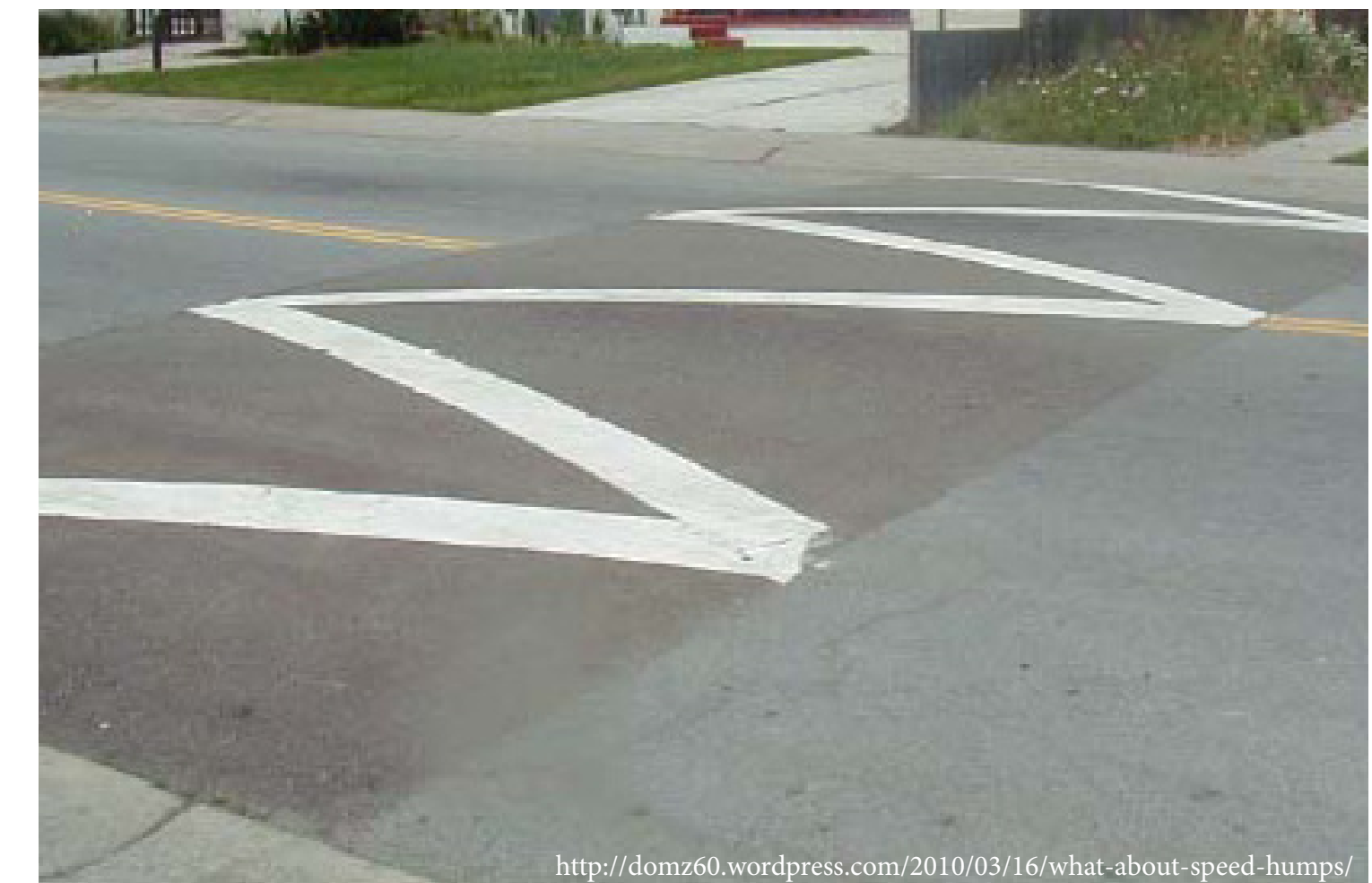
Raised tables slow traffic and allow snow plows to pass over
