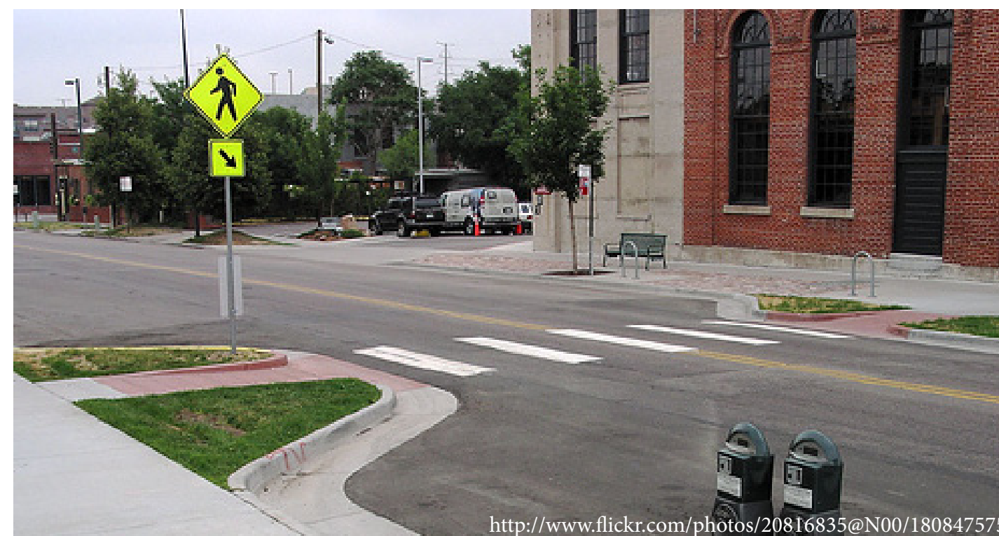
Bump outs slow traffic by narrowing the street, shorter street crossing
