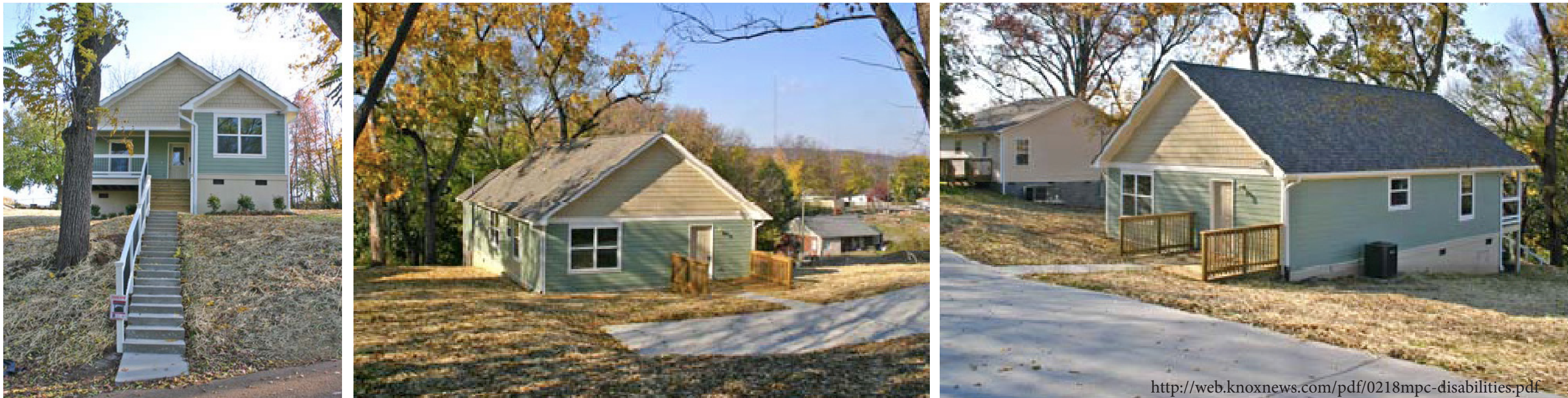
Above is an example of home modification from Knoxville, Tennessee. Prior to modification, the home was only accessible by a series of stairs. Moving towards visitability, a level, no-step entrance was added at the side of the house. Interior modifications included widening of doorways and installation of grab bars.
