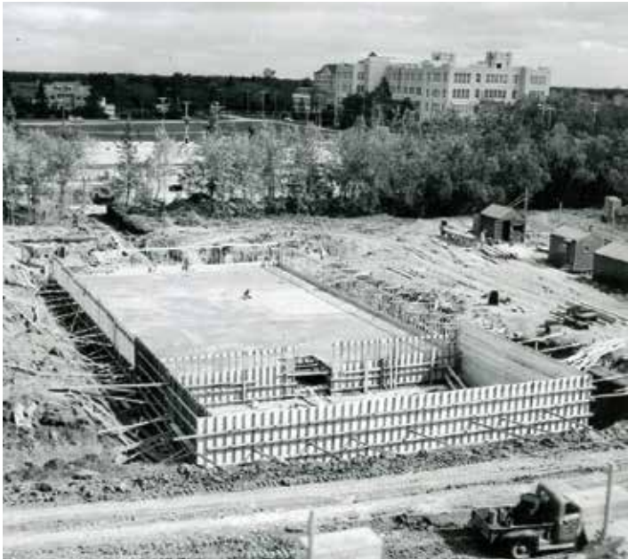
Fig. 8. Construction in progress.
