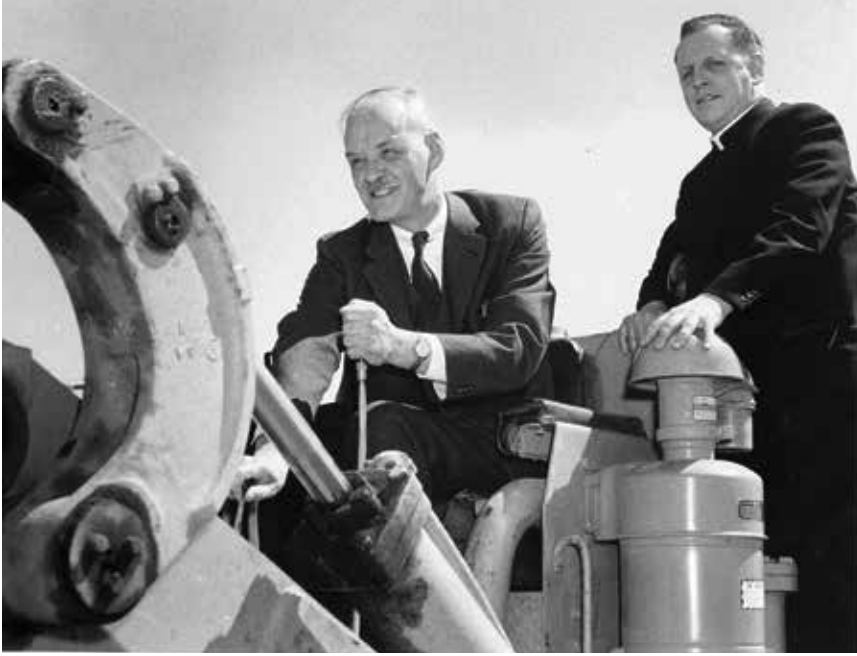
Fig. 6. Rector Ryan and University President Saunderson initiate construction of the new facilities on the U of M campus.
