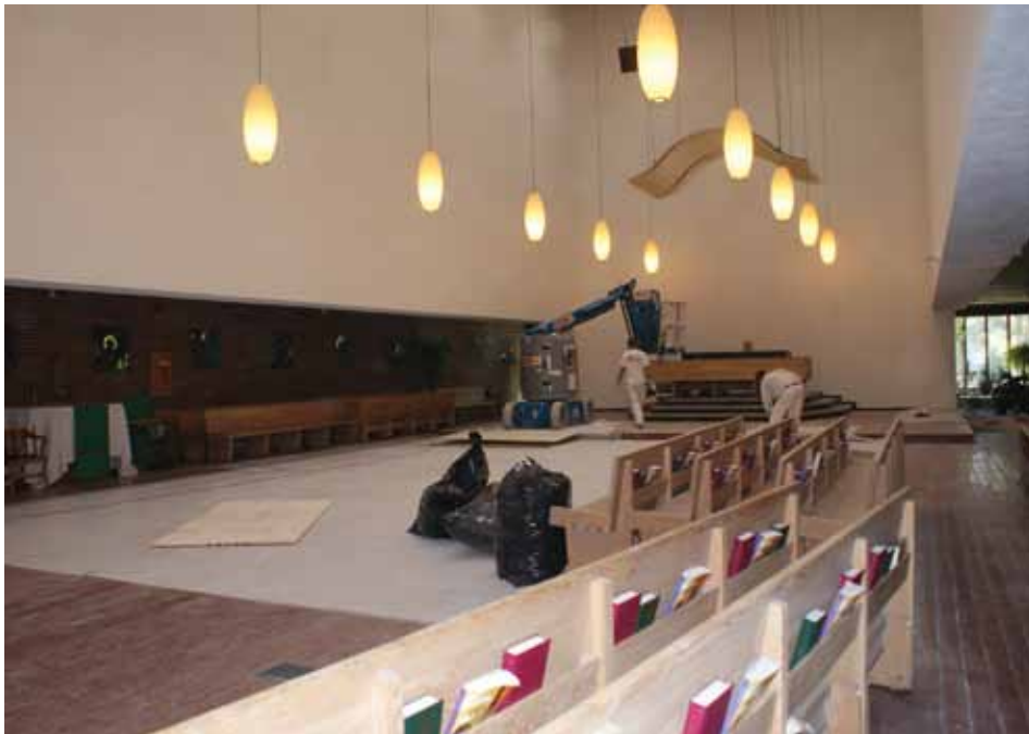
Chapel during the renovations
